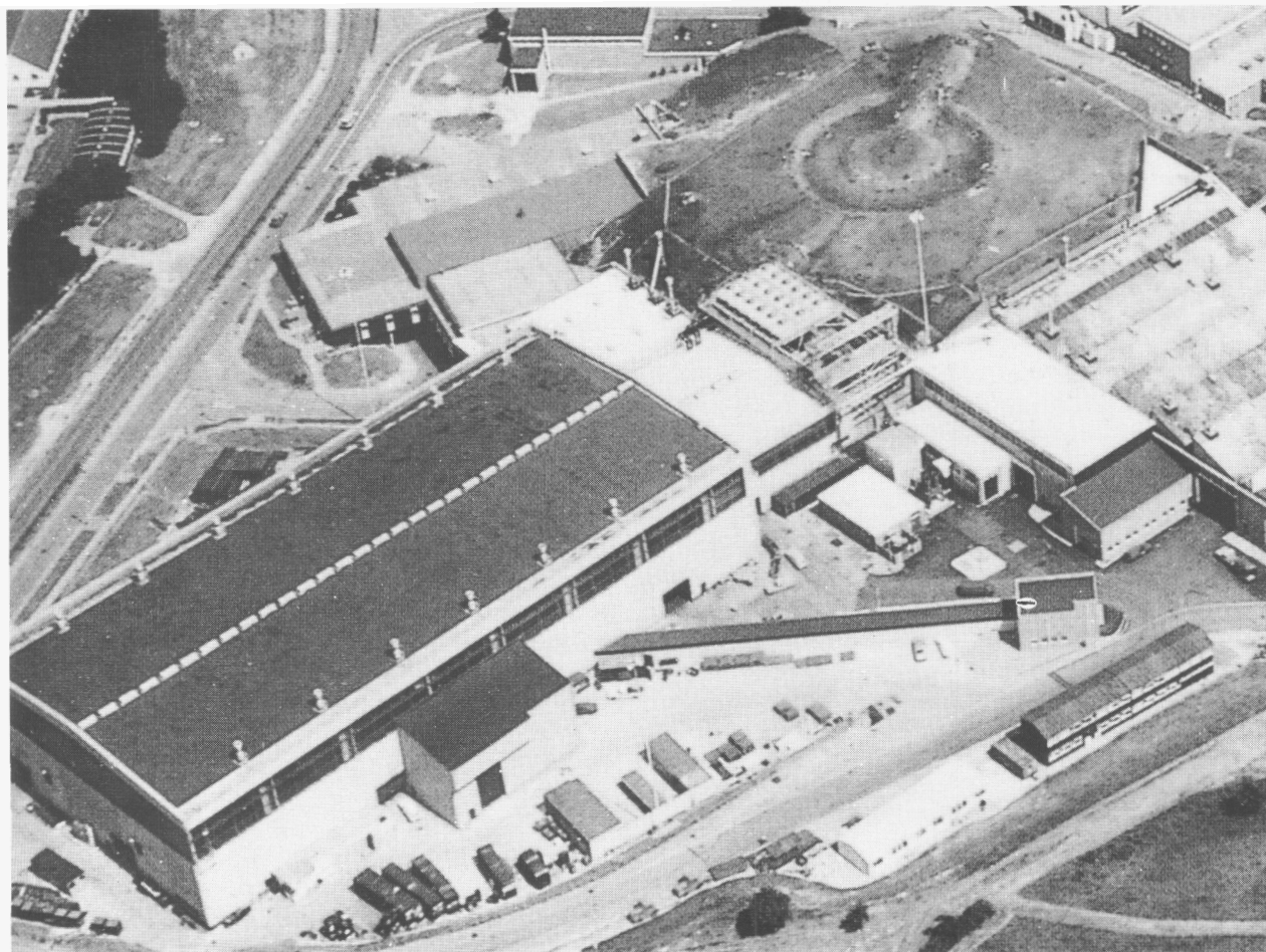
The spallation Neutron Source, ISIS, at Rutherford Appleton Laboratory. A long neutron channel, seen somewhat below and to the right of the centre of the photo, connects the diffractometer, in the smaller building, to the neutron source.
