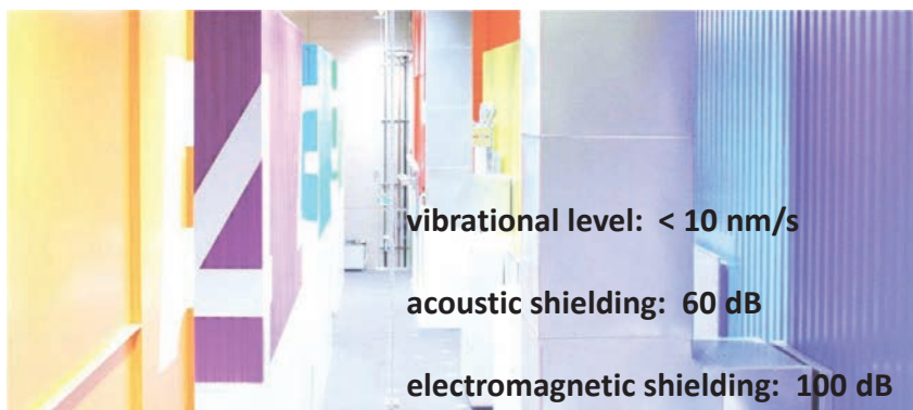
Fig. 7: Precision Laboratory (PL) at the MPI for Solid State Research in Stuttgart. The PL is a large isolated experiment hall partially enclosed by an office/service lab wing. The hall comprises eleven individually decoupled experiments. Each experiment is seismically, acoustically, and electromagnetically shielded from the environment. In order to technically realize these experimental environments, the challenges in the construction of the new laboratory pushed the technical limits and set new standards. A concrete box with a 60 dB attenuation encapsulates each experiment to acoustically isolate it from the immediate laboratory environment. External vibrations are dampened by a massive concrete block inside the acoustic box weighing between 100 t and 190 t. Set on air springs, vibrations are reduced to a level of <10 nm/s, several orders of magnitude smaller than the best industry standard today. For experiments operating at temperatures below 100 mK, the acoustic boxes are electromagnetically shielded by a closed metal shell yielding 100 dB attenuation. Further, the building has been constructed such that the general noise sources have been reduced as well. This includes, but is not limited to separate acoustic boxes at each experiment for noisy equipment, such as roughing pumps, shielded power lines, all optical data network and correspondingly all optical voice-over-IP telecommunication.
